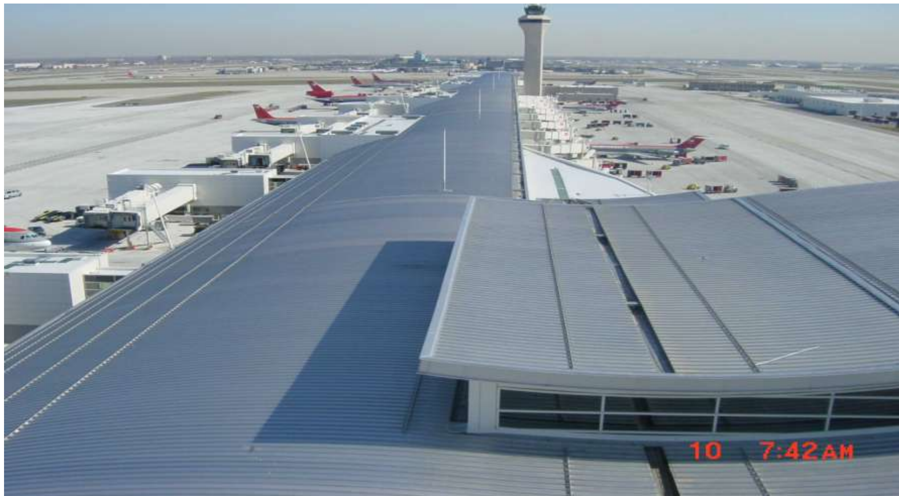
Detroit Midfield Terminal - USA
