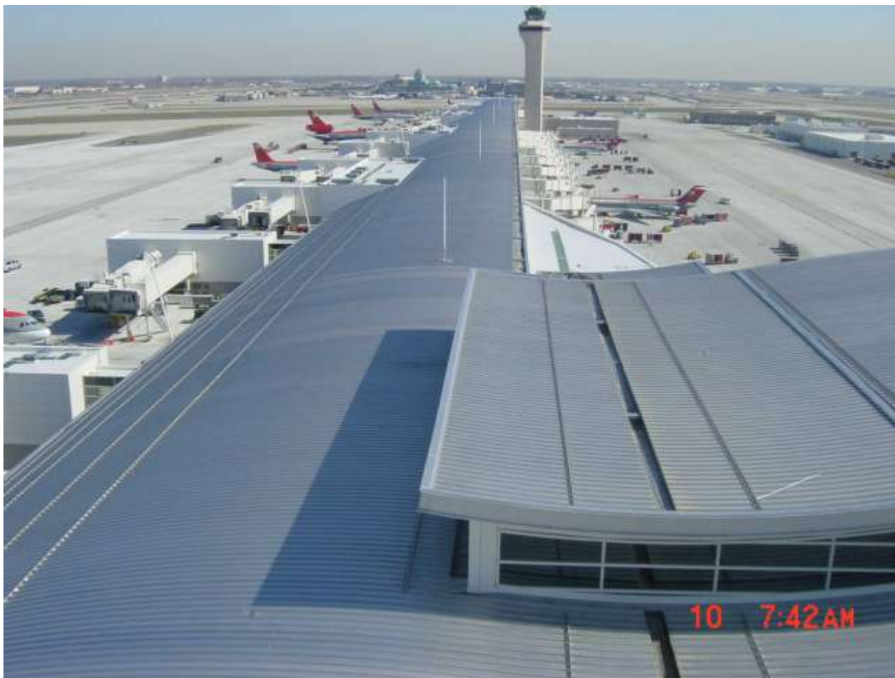
Detroit Midfield Terminal - USA
